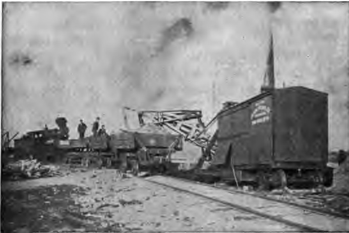
A modern excavating machine.
